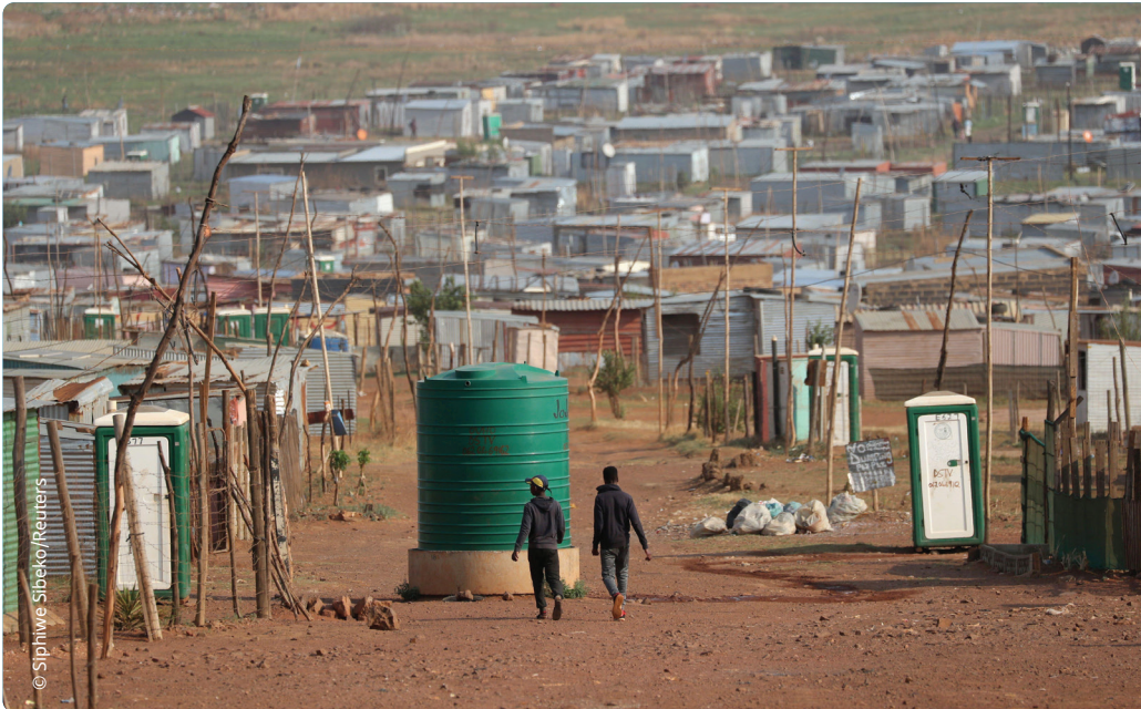
Water tanks at Lawley informal settlement near Johannesburg in the Gauteng province.
