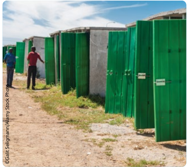
▲ Communal toilets in Langa in Cape Town, Western Cape province.
