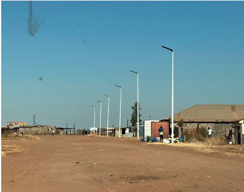
Figure 4: Doornkop solar powered streetlights
